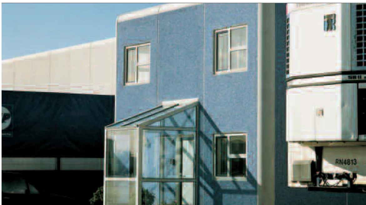
The entrance to the forwarding agency company HST Padborg, Denmark with prefabricated concrete elements with Collux® 8-12 mm dark blue.
